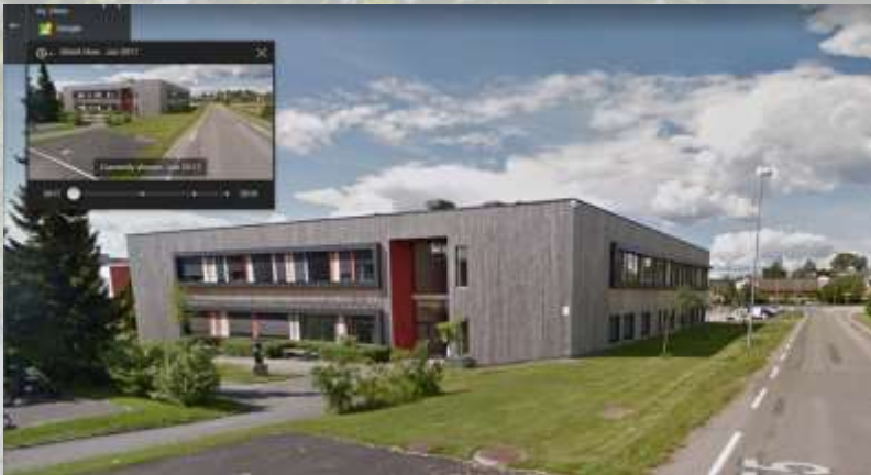
Figure 1: Mapping images of timber clad building having weathered and aesthetically changed. (CLICKDesign)
