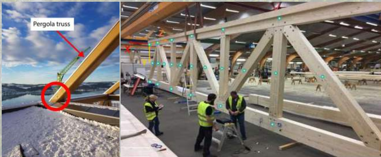
Figure 2: Accelerometers placed on the pergola of the Mjöstornet building in Norway (NTNU) and measurements on a glulam truss in Sweden (LNU and RISE).
