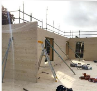
Figure 10. Assembly of the external wall panels (IsoTimber + CLT) and the intermediate floor panels (CLT). © Gustab AB.
