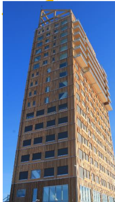
2019 18 storeys Glulam trusses Mjöstornet, Brummundal
