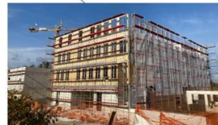
InnoRenew, 4 stories, CLT elements
