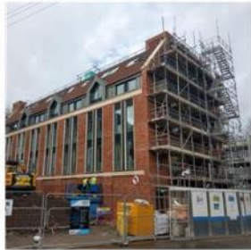
Trinity College building, 4 stories, CLT elements
