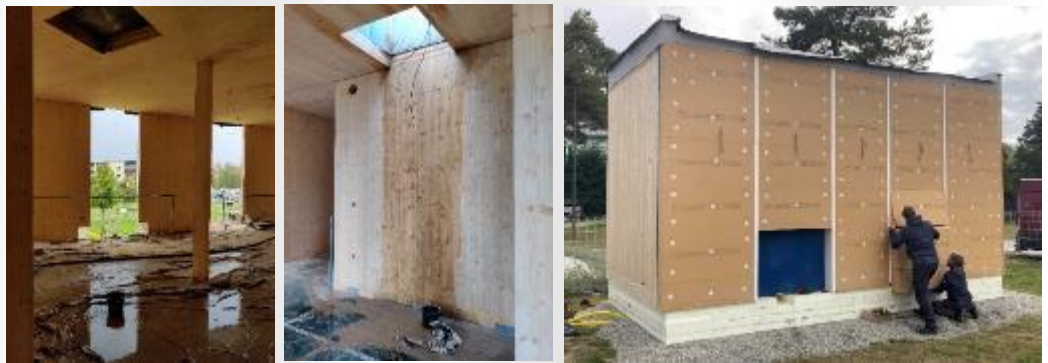
Pictures: Illustrating the importance of moisture safety during the construction phase. Left & centre: Rainwater ingress; Right: Installation of WoodLCC test house. ©WoodLCC
